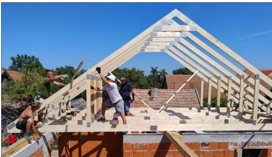
There they are erecting the roof trusses on the house. Silvester has helped throughout the construction period.
