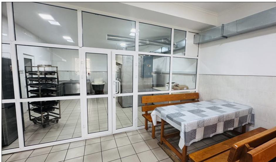
The wall behind the dining tables and the bakery, which can be seen in the background, will be demolished to make way for a community hall and dining room with a cooking kitchen.
