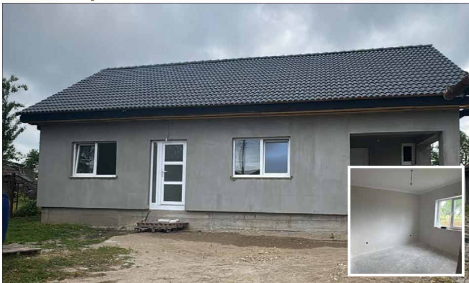
A good bit of progress. The house has now had its exterior refacing. Then it will be painted on the outside. One of the rooms inside the house.
