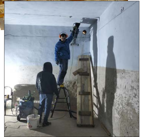
During the fall, holes were drilled in various places in the building for ventilation.
